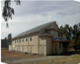
Assembly Hall, former Bonegilla Theatre, from the north-west
