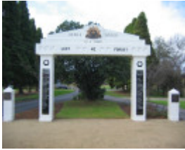
29405 Memorial Arch 1 Walnut Street Whittlesea 25
