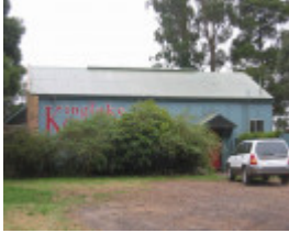
RSL Hall (Former)
