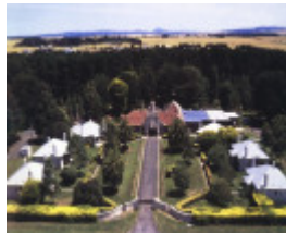
Rockbank Beam Wireless Station
