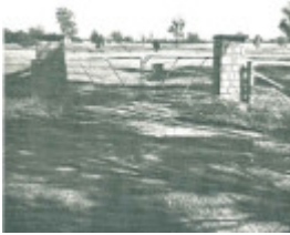
Gateway to Murchison camp 13, built by Italian labour c1944.
