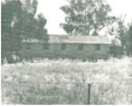
Former internment camp hut, off River Road, Murchison
