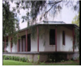
1 byramine homestead front view homestead
