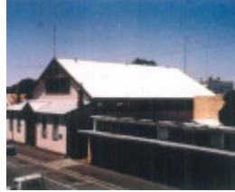
Mont St. Quentin Barracks, 1990
