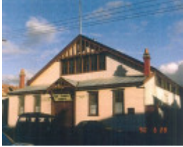
Mont St. Quentin Barracks, 1990
