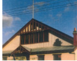
Mont St. Quentin Barracks, 1990
