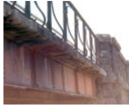
Road Over Railway Riddells Creek
