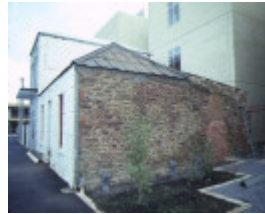
cottages hargreaves street bendigo side view specimen cottage jul1984
