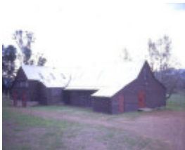
h00371 murrindindi station melba hwy yea woolshed she project 2003
