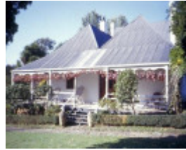
h00371 1 murrindindi station melba hwy yea homestead north elevation she project 2003
