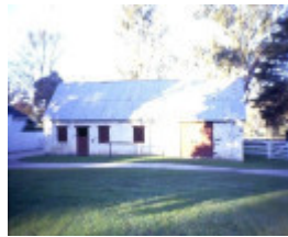
h00371 murrindindi station melba hwy yea stone stables she project 2003
