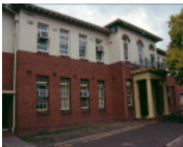
h02031 preston tramway workshops admin building may03 aj
