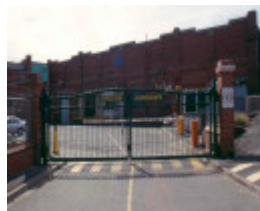
h02031 preston tramway workshops entry gates may03 aj
