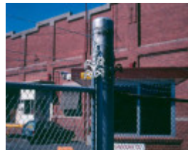
h02031 preston tramway workshops fence detail may03 aj
