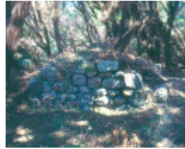
H02019 sealers cove saw mill stonework
