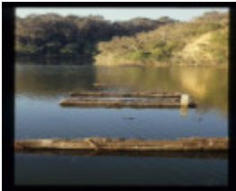
LAKE TYERS TIMBER COMPANY TRAMWAY BRIDGE
