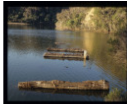
LAKE TYERS TIMBER COMPANY TRAMWAY BRIDGE
