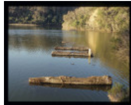
LAKE TYERS TIMBER COMPANY TRAMWAY BRIDGE
