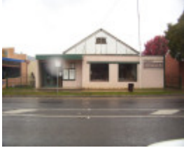
Rsl Hall & Flagpole, former
