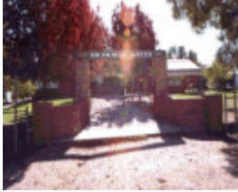
Chiltern Primary School Memorial Gates
