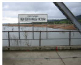
h00989 bethanga bridge bellbridge border jun20044 mz
