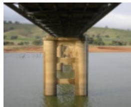
h00989 bethanga bridge bellbridge pylons 02 jun20044 mz
