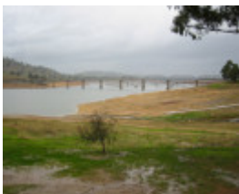
h00989 bethanga bridge south from vic 02 jun20044 mz
