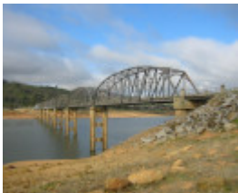
h00989 bethanga bridge bellbridge north nsw side jun20044 mz
