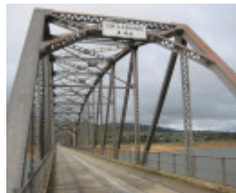
h00989 bethanga bridge bellbridge pratt truss north nsw 02 jun20044 mz
