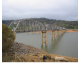
h00989 bethanga bridge bellbridge south side from nsw jun20044 mz
