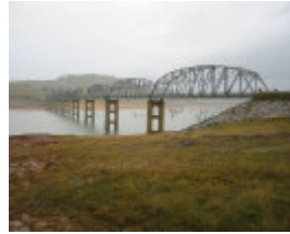
h00989 01 bethanga bridge south from vic 01 jun20044 mz
