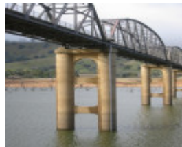
h00989 bethanga bridge bellbridge pylons 01 jun20044 mz
