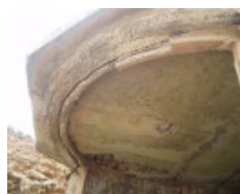
Fortifications, Point Lonsdale Road, Queenscliff
