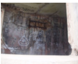
Fortifications, Point Lonsdale Road, Queenscliff
