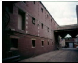
h02050 richmond maltings west elevation 1930 malthouse mz june03
