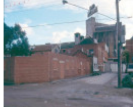
h02050 1 richmond maltings view along gough st ro jun03
