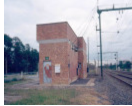
h02025 1 bunyip sub stationjul03 jc
