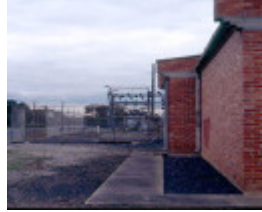
h02025 2 bunyip sub stationjul03 jc
