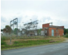
BUNYIP RAILWAY SUB STATION SOHE 2008
