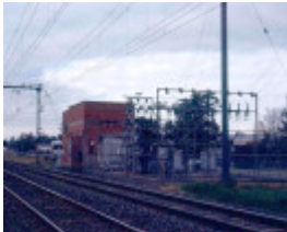
h02025 3 bunyip sub stationjul03 jc
