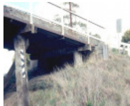
h02054 portland flat road bridge south abutment 0903 mz
