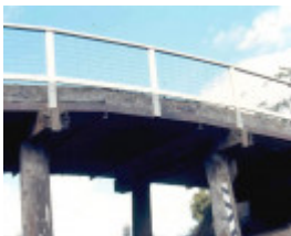
h02054 portland flat road bridge west ele centre span 0903 mz
