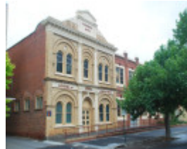
FORMER MECHANICS INSTITUTE AND SCHOOL OF MINES SOHE 2008
