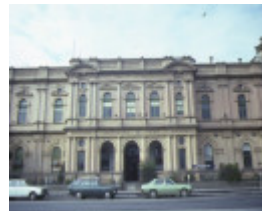
former sandhurst mechanics institute bendigo entrance jul1984
