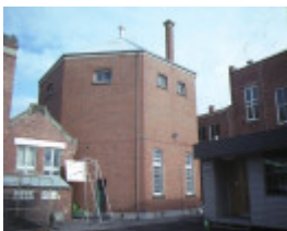
former sandhurst mechanics institute bendigo rear view jul1984
