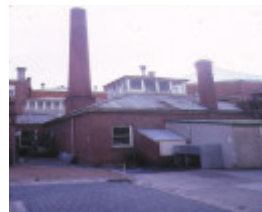
former sandhurst mechanics institute bendigo workshops aug1983
