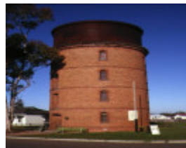
1 former railway water tower comyn avenue murtoa front view
