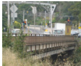
h00050 hawthorn bridge may 05 view east
