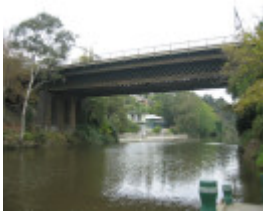
h00050 1 hawthorn bridge may 05
