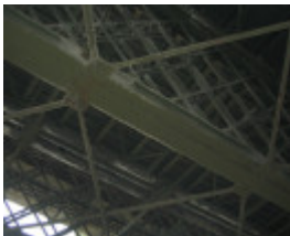
h00050 hawthorn bridge may 05 trusses
