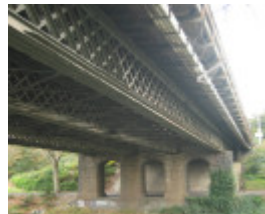
h00050 hawthorn bridge may 05 view from below
