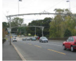
h00050 hawthorn bridge may 05 roadway
