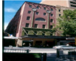
h01542 1 fourth victoria building
