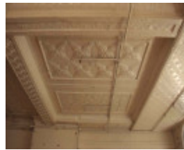
h01542 fourth victoria building wunderlich ceiling
