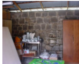
h02071 portland inn bluestone wall
