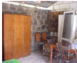
h02071 portland inn bluestone wall 2
