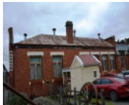
CMP Tech Addition north elevation (Source: CMP, 2021)
