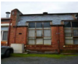
Former Art department, glazing detail, north elevation (Source: CMP, 2021)
