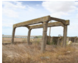
13045 marshall pipe works3
