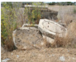
13045 marshall pipe works4
