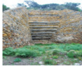
BELL POINT LIME KILN SOHE 2008
