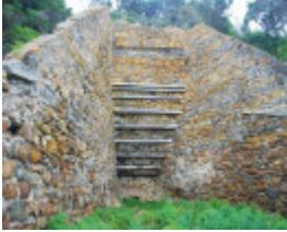
BELL POINT LIME KILN SOHE 2008
