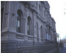
law courts bendigo facade detail jul1984
