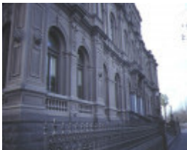
law courts bendigo facade detail jul1984
