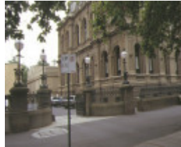
law courts bendigo entrance gates jan1999
