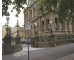
law courts bendigo entrance gates jan1999
