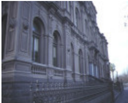
law courts bendigo facade detail jul1984
