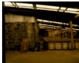
Sunnyside Wool Scour Interior
