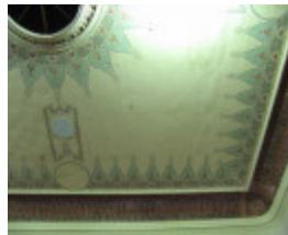
Town Hall_Maryborough_painted ceiling in main hall_7 Nov 07- KJ
