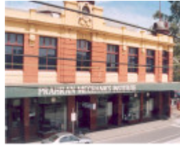
h00400 1 facade full
