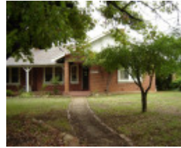
h01065 holy trinity anglican cathedral precinct wangaratta armstrong house 41 ovens st 2005
