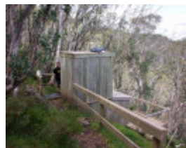
h00046 gantner hut the third toilet feb2005 as 011
