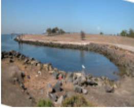
Power Station Park Seawall Williamstown March 2003
