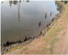
Jack's Magazine Canal And Wharf Maribyrnong July 2003 001
