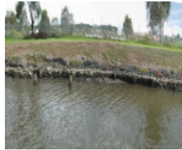
Jack's Magazine Canal And Wharf Maribyrnong July 2003 003
