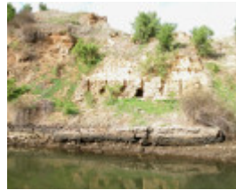
Maribyrnong Sand Company Jetty And Tramway Loading Chute Maribyrnong May 2003 002
