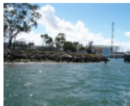
Channel Deepening Project
