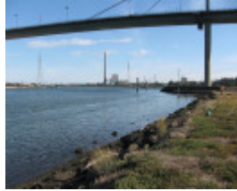
Channel Deepening Project
