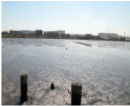
Stony Creek Pier Piles Maribyrnong March 2003 001
