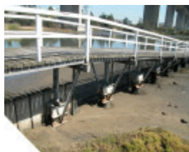
Stony Creek Wharf 2 Maribyrnong March 2003 Concrete Sheet Piling And Wharf 2
