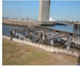
Stony Creek Wharf Maribyrnong March 2003 Concrete Sheet Piling
