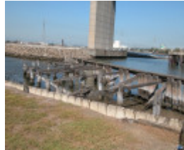
Stony Creek Concrete Sheet Piling Maribyrnong March 2003 003
