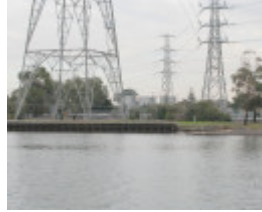
Newport Oil Wharves Williamstown June 2003 003
