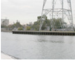
Newport Oil Wharves Williamstown June 2003 001
