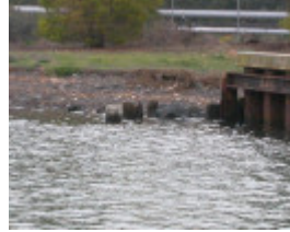
Newport Oil Wharves Williamstown June 2003 002
