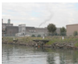
Commonwealth Fertilisers Wharves Maribyrnong July 2003 Wharf And Bollards
