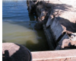
Footscray Bond Store Wharf Maribyrnong March 2003 Sheet Piling
