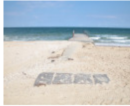
Harold St Drain Port Melbourne April 2006 003
