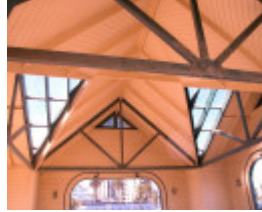
St Kilda Pier Port Melbourne April 2003 003
