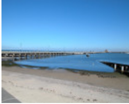
St Kilda Pier Port Melbourne April 2003 001
