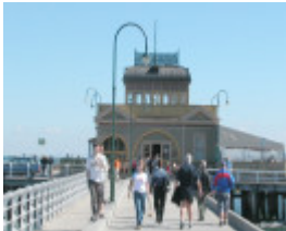
St Kilda Pier Port Melbourne April 2003 004
