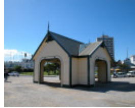
St Kilda Pier Port Melbourne April 2003 002
