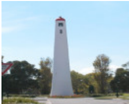
Port Melbourne Lead Lights And Access Jetty Port Melbourne July 2003 001
