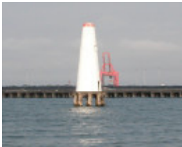
Port Melbourne Lead Lights And Access Jetty Port Melbourne July 2003 004
