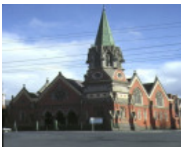
1 former congregational church ballarat front view aug1985
